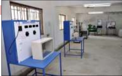
Laboratory Details / Thermal Engineering Lab - I
